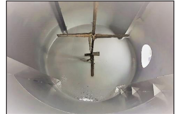
Tank interior after ARC S3 application.
