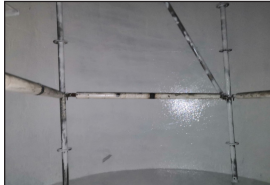
ARC S3 applied to interior of carbon steel tank.
