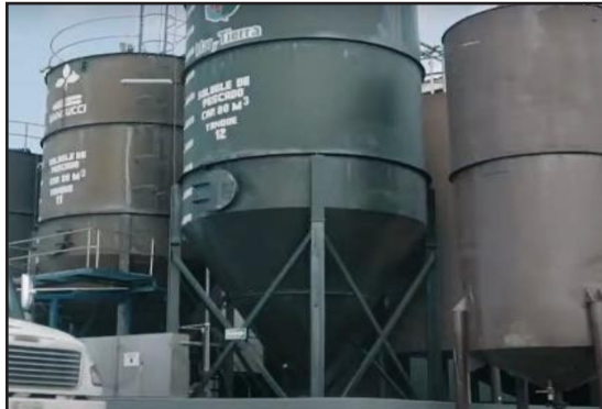
Liquid fertilizer storage tanks before maintenance.
